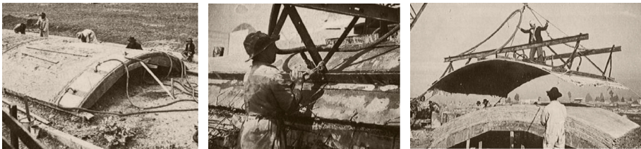
Fig. 4. A. View of the vacuum pump. B. Installation of the lifting system. C. Lifting of one of the shells. All in PROA Magazine no 71, 1953. Bogotá.
